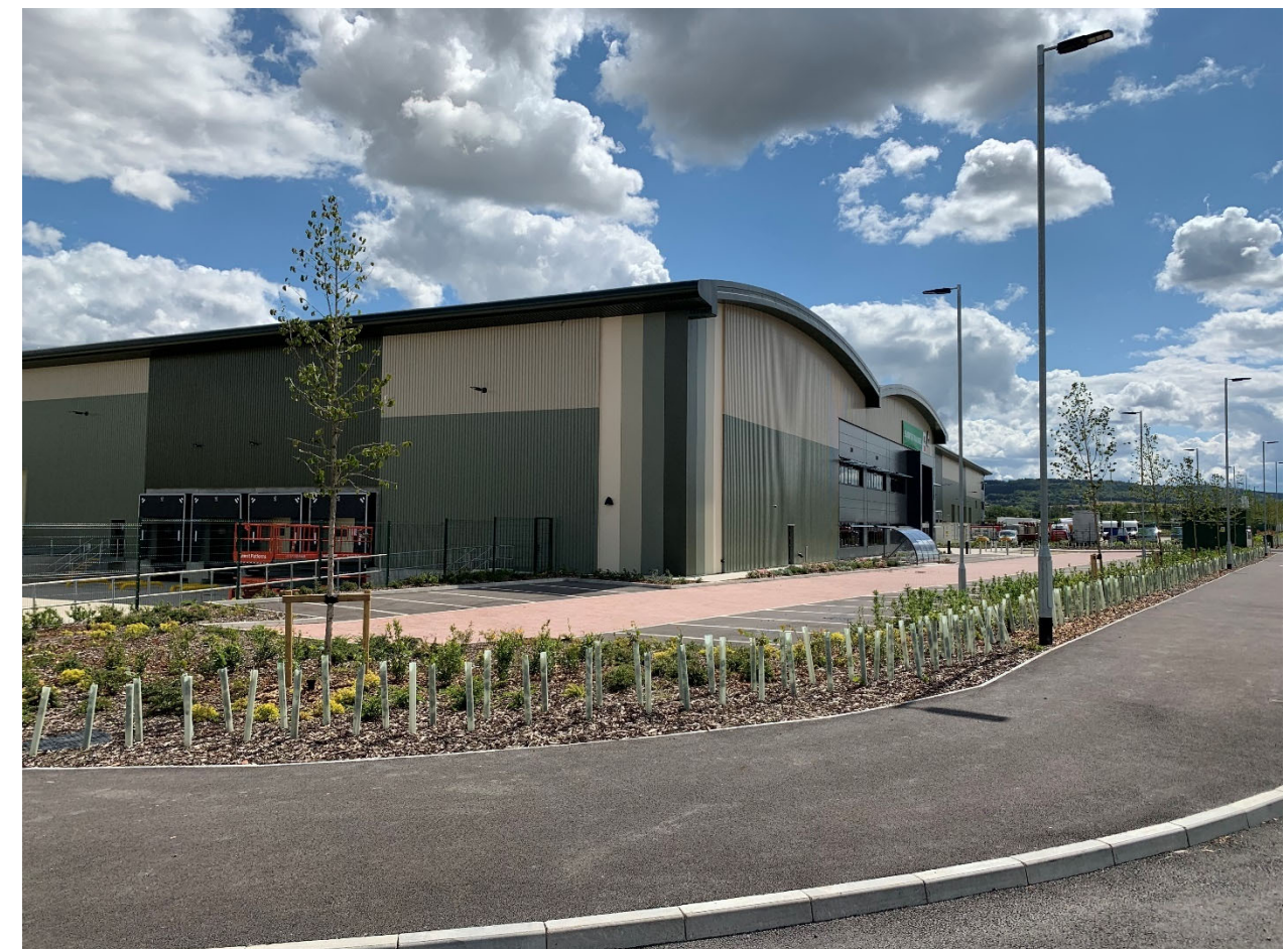
Fig 3649. Column mounted and building mounted, light fittings for the development plots and highways.
