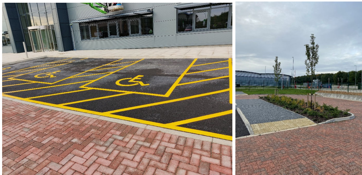
Fig 53. Accessible parking adjacent to main entrance, and crossing detail within car park.
