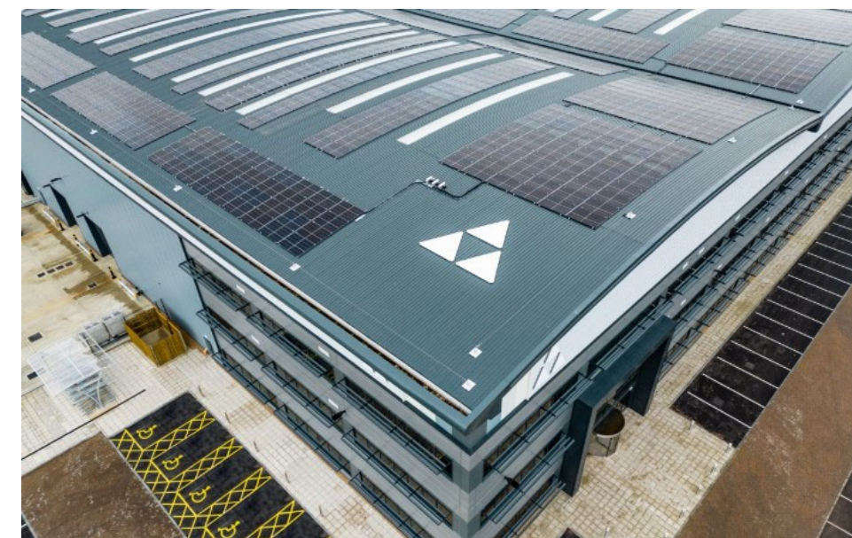
Fig 45. Illustrative example of a PV installation on the roof.
