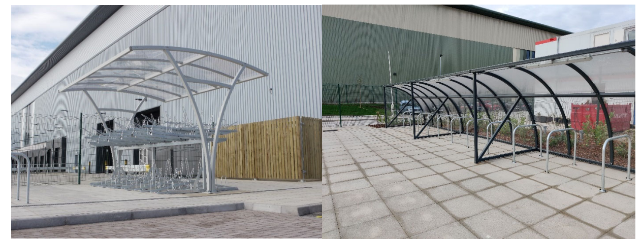
Fig 51. Examples of a secure and covered cycle shelter.
